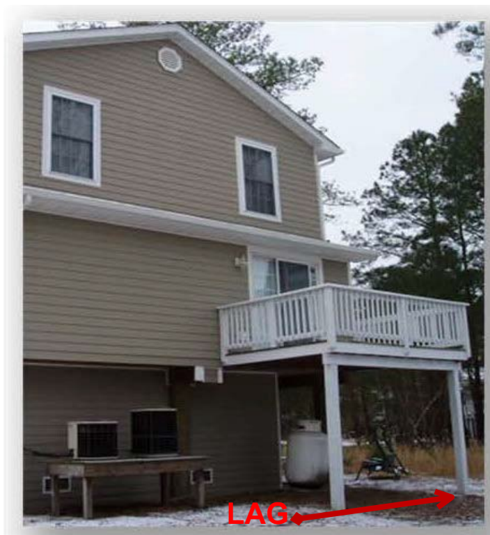
Figure 3: LAG - Structure with Attached Deck
