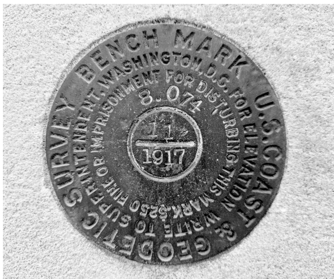
Tidal benchmark at Federal Courthouse (NAVD88 elevation is 7.57 feet).
